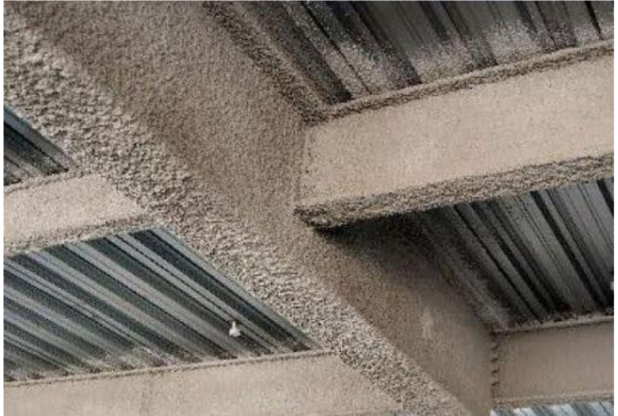
Photo: example of sprayed vermiculite
